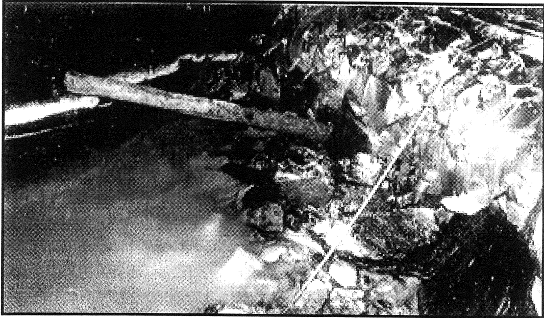
Figure 5 - Debris jammed into head of Miner
